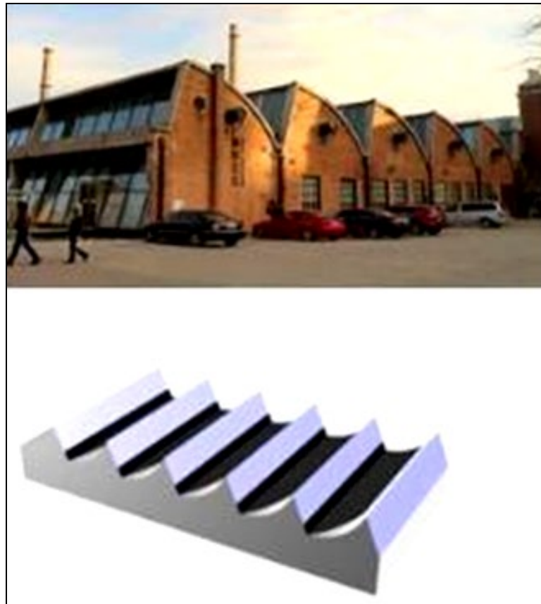
Fig 2: North-Light/Saw-Tooth Roof
